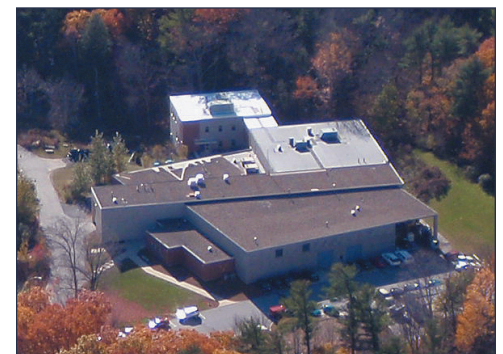
Aerial view of Chase with the new addition. Photo courtesy of Rob Roseen, UNH Stormwater Center.
