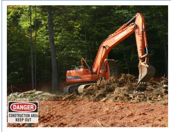
Construction on the new CCOM addition has begun!
