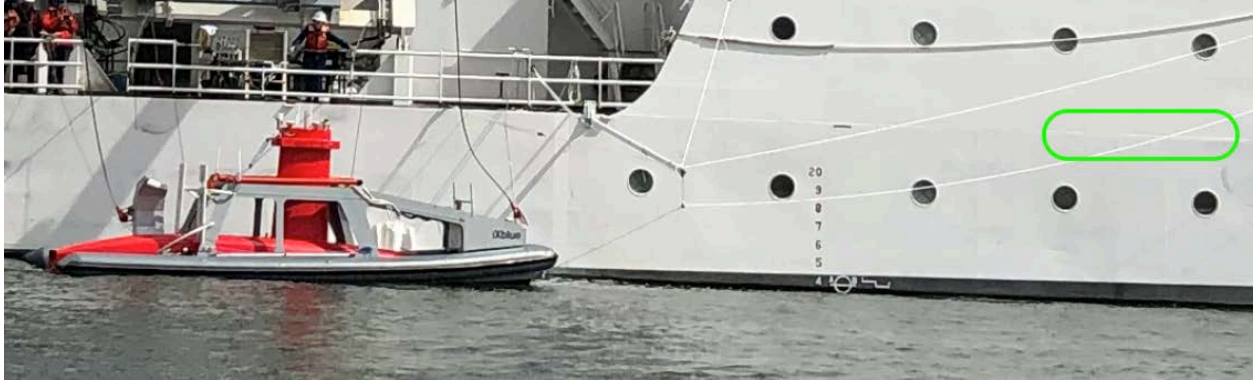
The painter boom installed forward of the Davit in 2019, and the preferred installation location marked in green.
