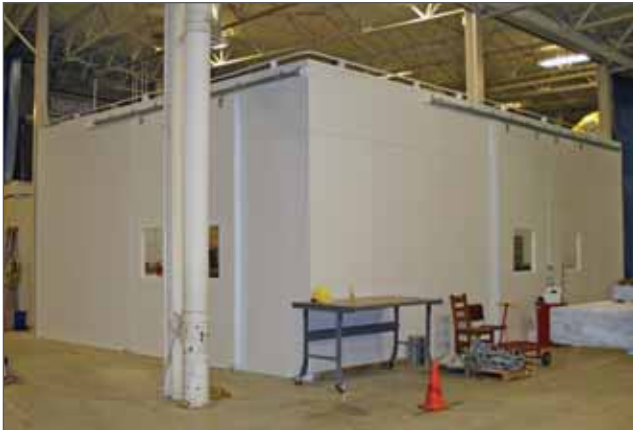
Figure 1-9. New room constructed in the high bay for ROV storage.
