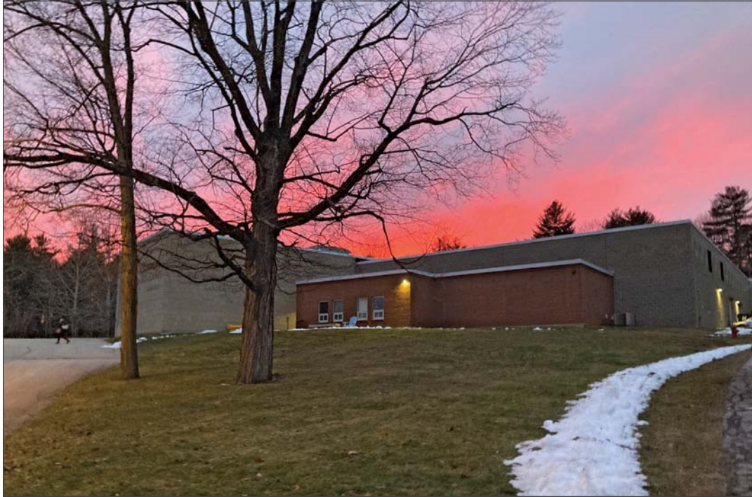
Figure ES-47. Sunset over the Center's home—the Jere A. Chase Ocean Engineering Lab on UNH's Durham campus.
