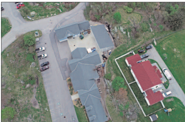
Figure I-10. The Pier Support Building at the UNH Coastal Marine Lab in New Castle, New Hampshire. Photo courtesy of Matt Pickett, Oceans Unmanned.
