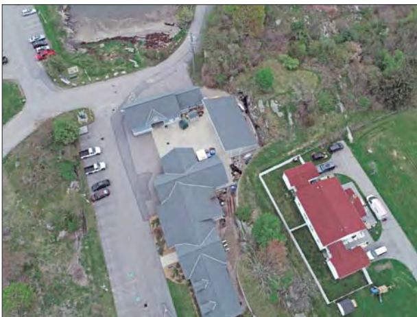
Figure I-9. The Pier Support Building at the UNH Coastal Marine Lab in New Castle, New Hampshire. Photo courtesy of Matt Pickett, Oceans Unmanned.
