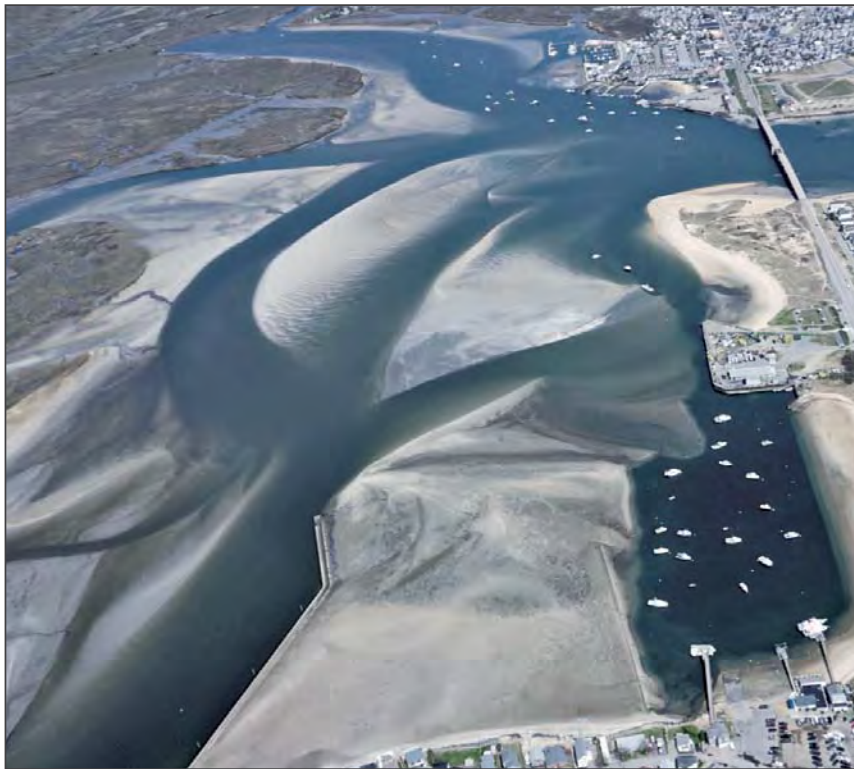
Figure 33-8. Aerial photograph of Hampton/Seabrook Harbor taken in 2017 showing the channel cuts across the middle ground (flood tidal delta) and infilling of the navigational channel leading to a large portion of New Hampshire's fishing fleet.
