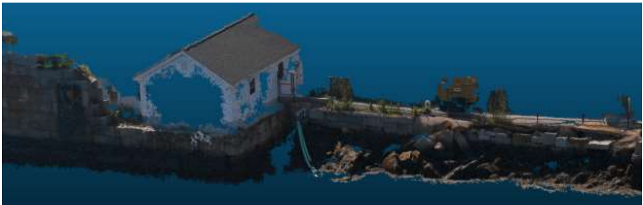
Figure 44-10: Color point cloud of Fort Constitution waterline.
