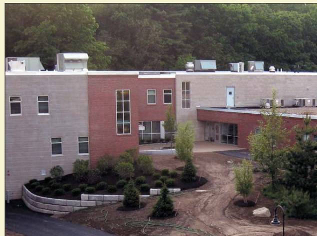
The 10,000 square foot addition, completed in 2008.
